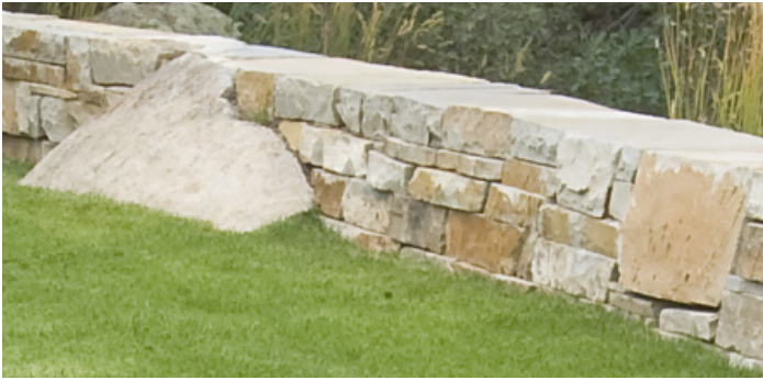
Above (Option 1): Dry stacked sandstone. In the example large boulders are integrated with smaller cleft blocks.
